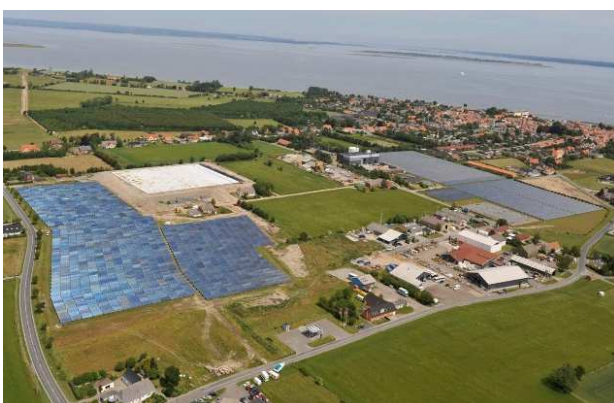
Picture of the large-scale solar plant and the large heat storage tank with foil cover and the biomass heating power plant in Marstal (DK)
