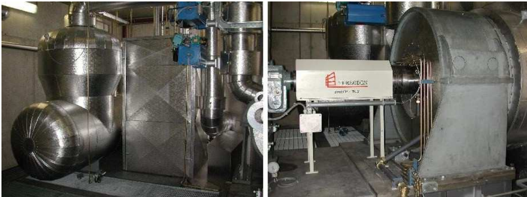
Picture of the ORC plant and the turbine - Lienz biomass CHP plant
