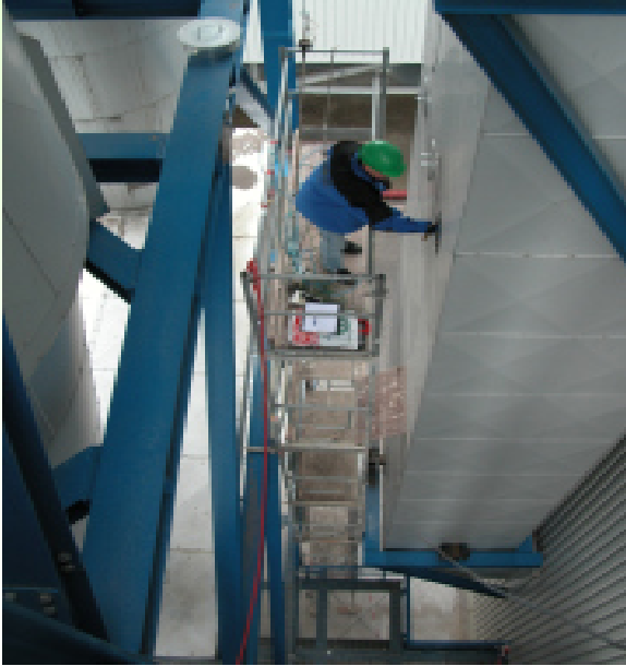
Measurement campaign at a real-scale combined heat and power plant
