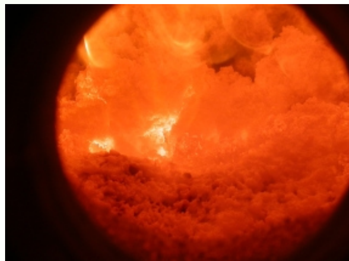
View into the furnace of a pilot-scale grate fired combustion plant during a test run
