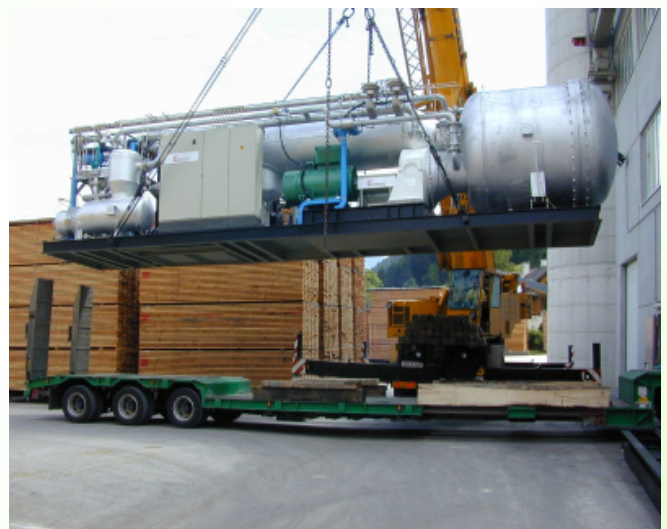
ORC module in container design (400 kW el ) at its delivery at the CHP plant
